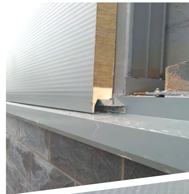
Joint with gap for horizontal application
