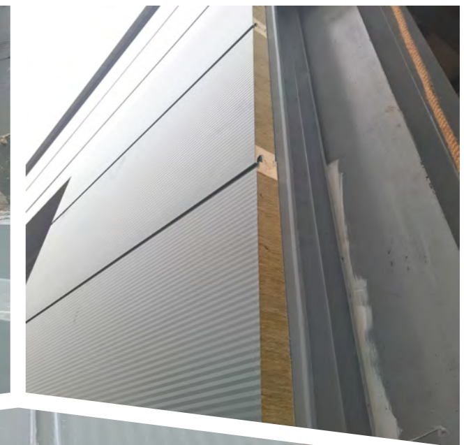
Joint without gap for horizontal application
